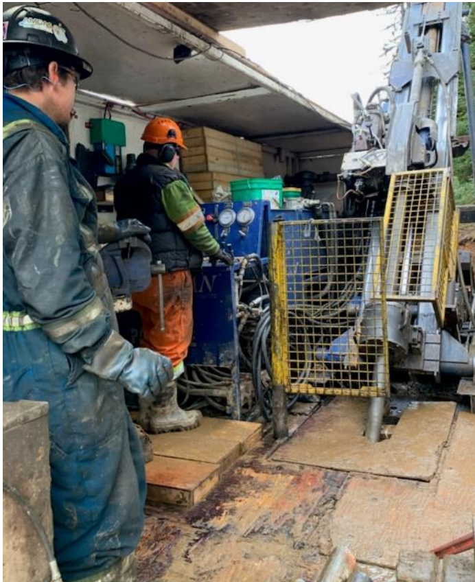
Figure 3. Drillers in action during the 2021 program.
