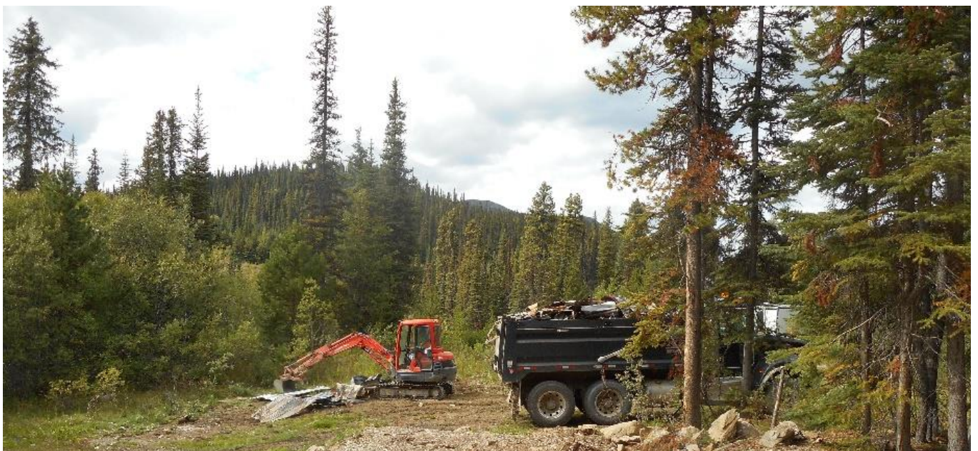
Figure 11. Heavy machinery at work to reclaim a Cassiar North site
