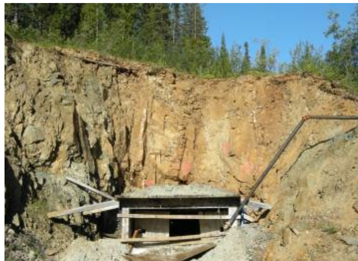
Historical Taurus Underground Portal
