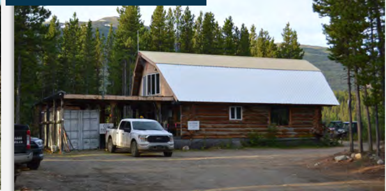
48-PERSON CAMP with Grid Power & Water
